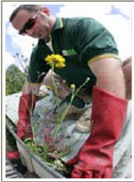
Once the gutters are free of debris the fitter will lay the mesh over the gutters and lower part of the roof, securing the mesh to the gutters with colourbond trims.
